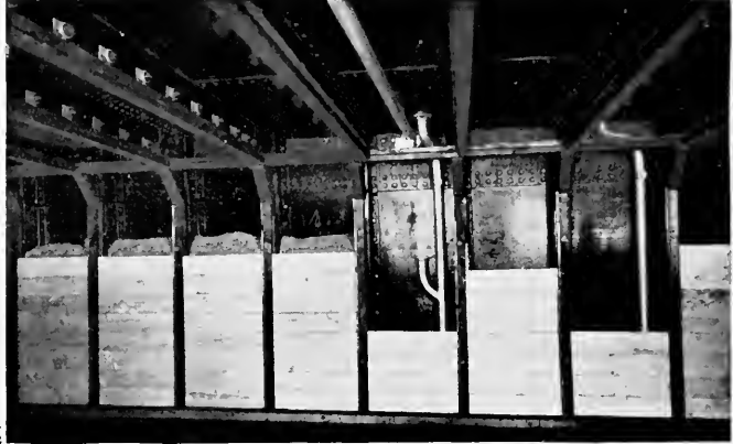
Photo shows how a 'tween deck section is insulated.
